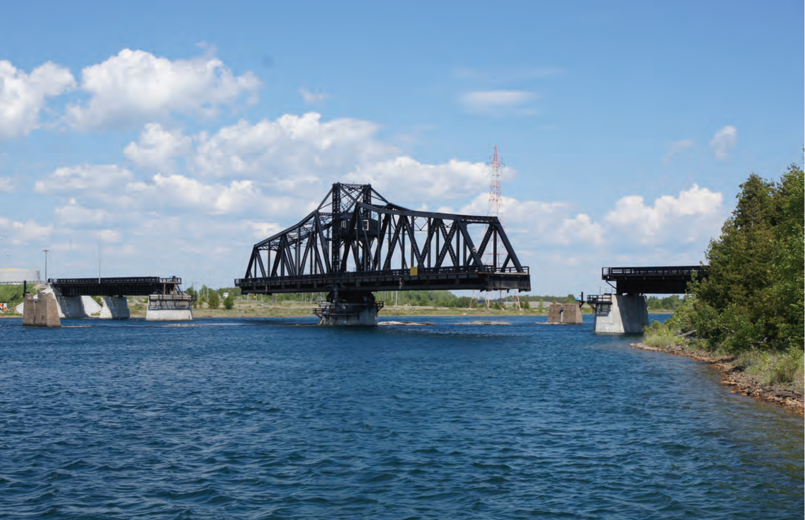
▲ The Heritage Swing Bridge that joins Little Current to the mainland gave us a display. The bridge will have its 100th anniversary in 2013.
